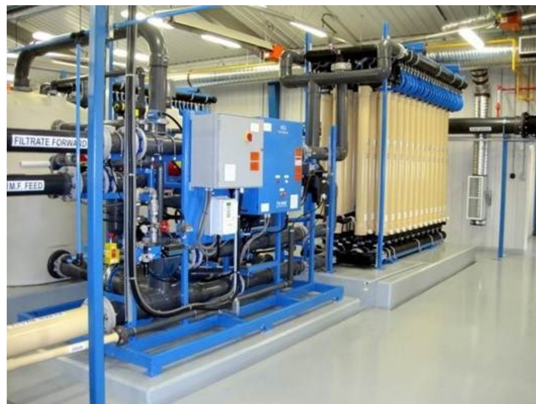
Typical Pressurized Ultrafiltration Membrane Package Treatment Plant
